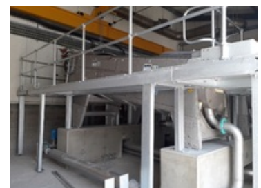
Installation photos of HUBER Screw Press Q-PRESS® at Plymouth Central
