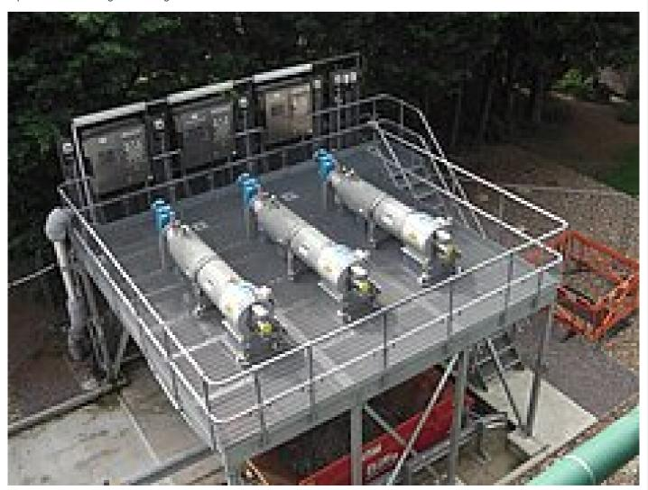
These new improvements in its design meant that the STRAINPRESS® was now suitably upgraded to ensure that the whole life cost of the unit was reduced and thus allowed it to comply with the latest specifications and market requirements.
