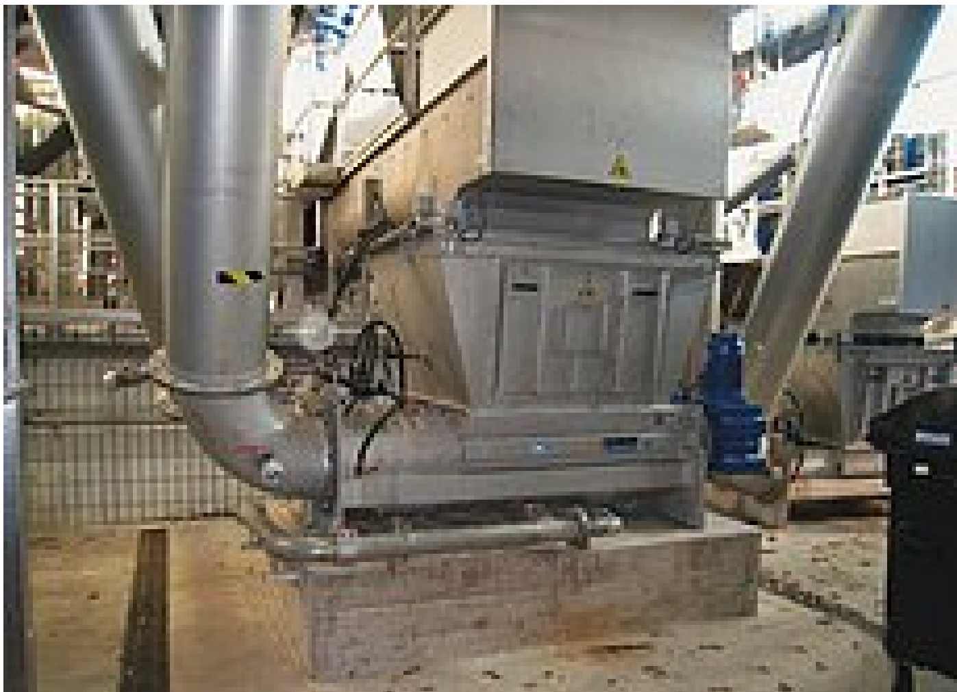
HUBER Wash Press WAP@ 2x8 with 16m³/h throughput each
