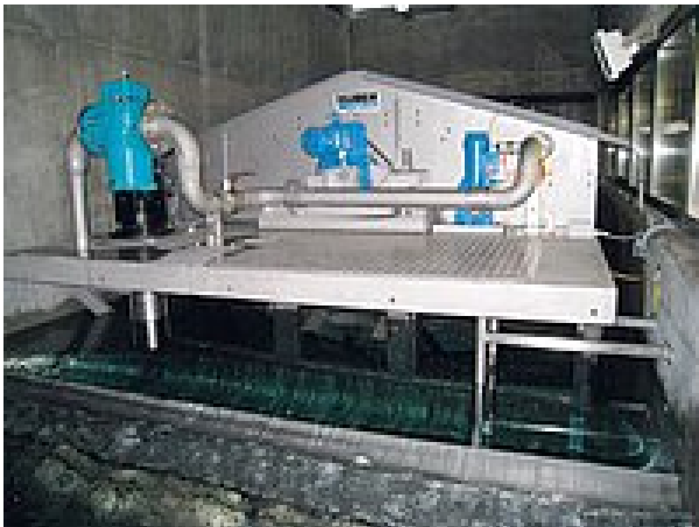
RoDisc® Rotary Mesh Screen installed in the inlet structure from where a 10 km long pipeline runs to the water works
