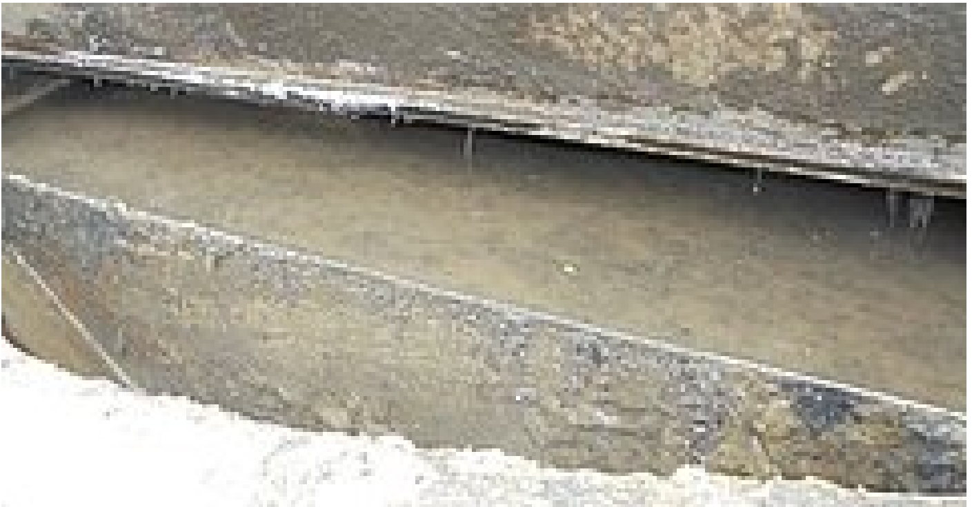
Figure 2 – Organic-rich wash water returned to the feed
