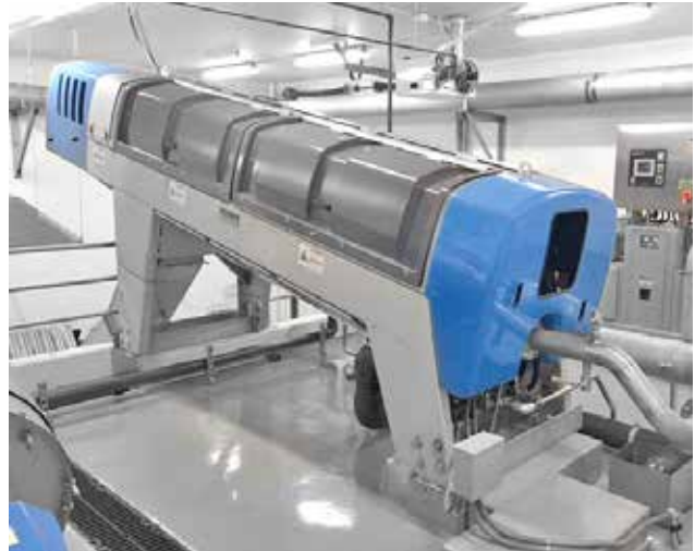
Q-PRESS® 620.2 for surplus sludge dewatering.
