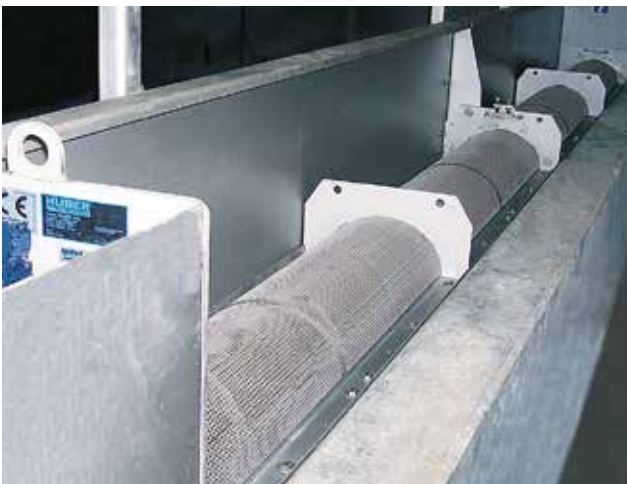
View of the downstream side of a HUBER Storm Screen ROTAMAT® RoK2.
