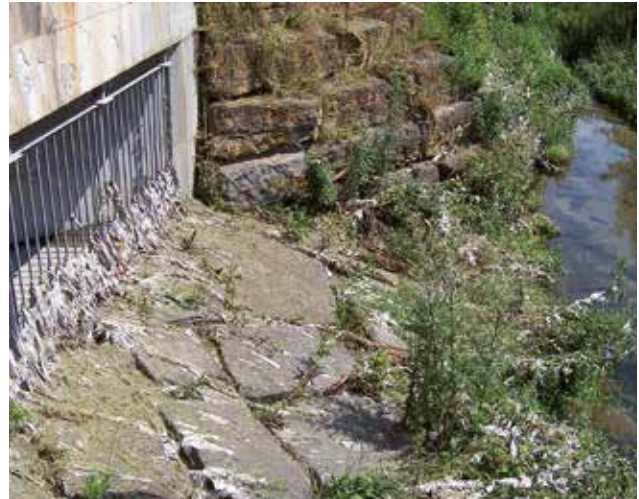
Unsightly matter discharged during storm events, typical for stormwater discharges without coarse material retention.
