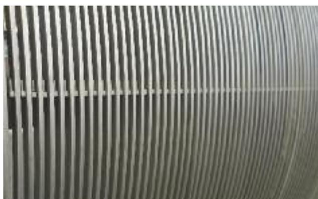
*The rake tines, fully engaging with the bar rack, prevent jamming of solids in the bar spacings.*
