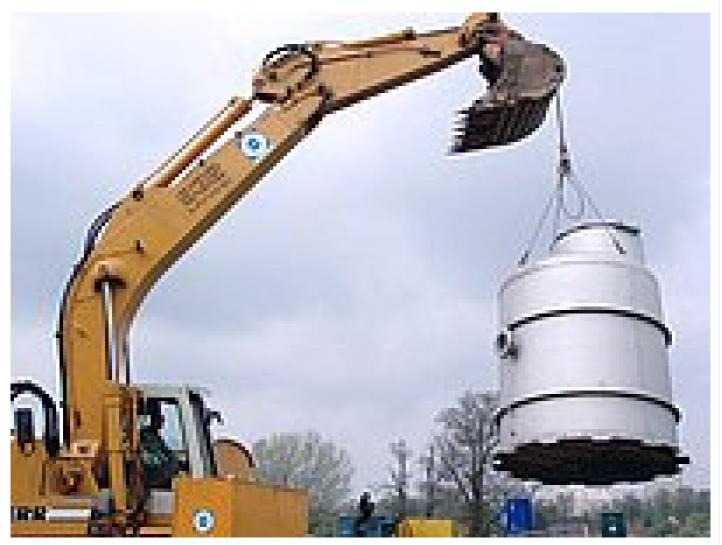
Prefabricated manhole, completely made of 1.4307 (AISI 304 L) stainless steel, watertight, with entrance and installation opening in accordance with DVGW sheet W122.
