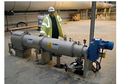
STRAINPRESS® installation on mezzanine floor
