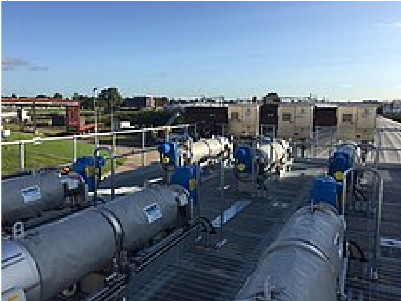
Minworth STW STRAINPRESS® Installation
