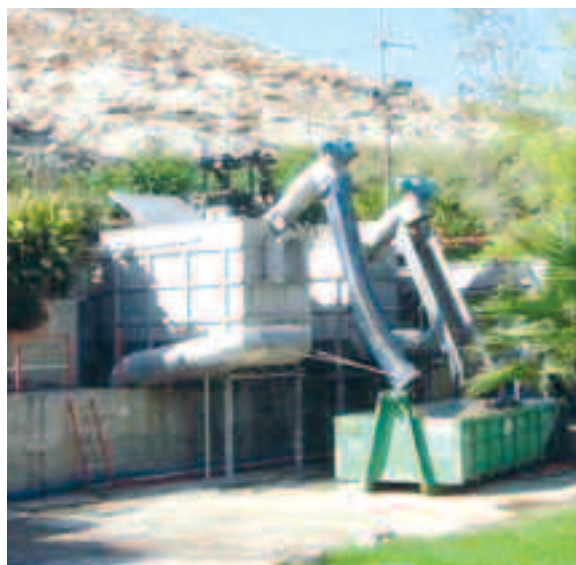
ROTAMAT® Fine screens installed in the Middle East ...
