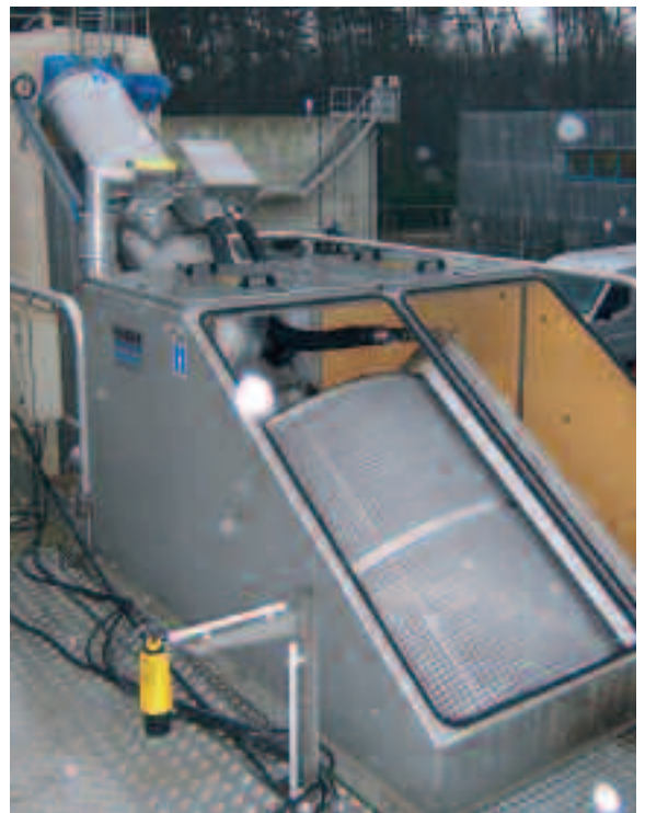
Micro-Screen ROTAMAT® RoMem in a channel
