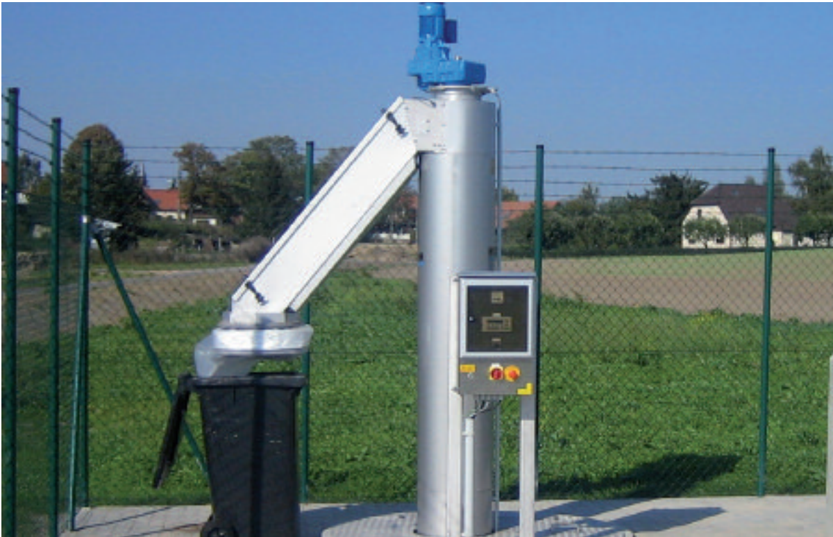
Outdoor installation of a ROTAMAT® Screen for pumping stations RoK 4
