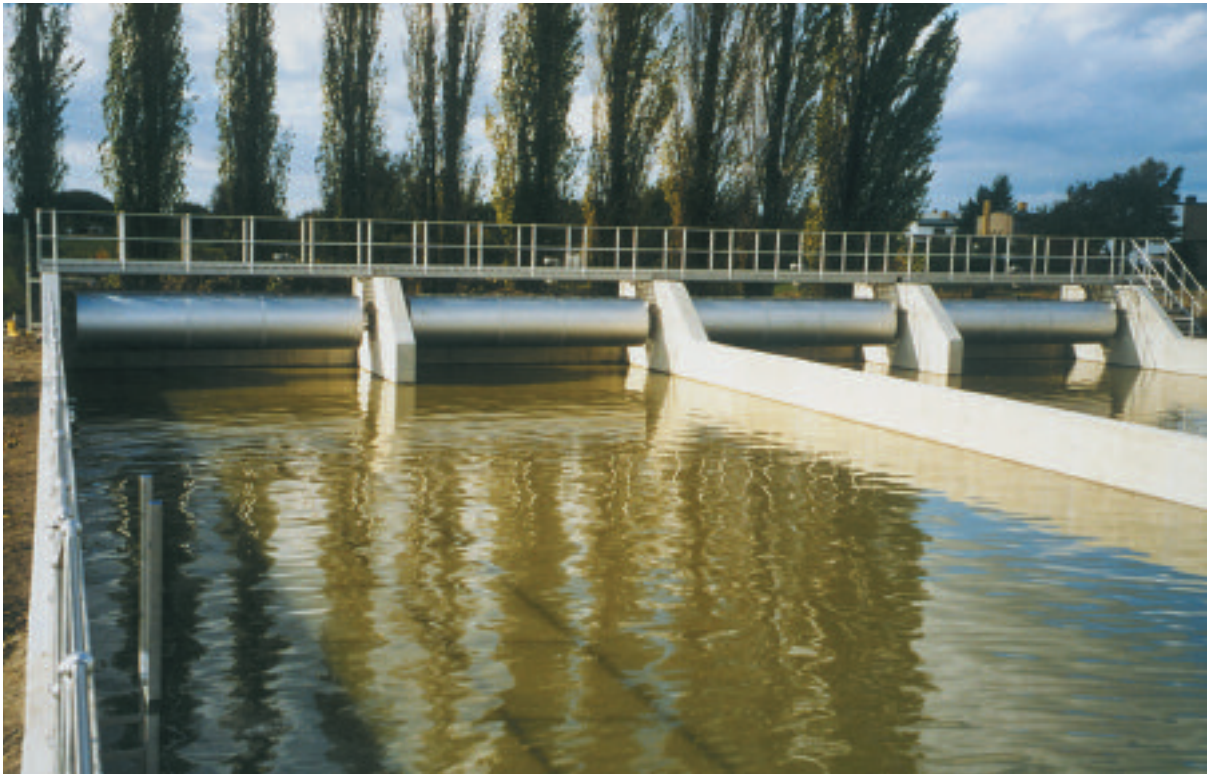
HUBER Tipping Buckets SK for efficient stormwater storage tank cleaning
