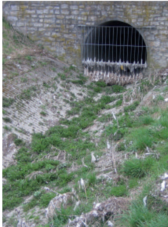
Stormwater overflow structures without a preceding fine screen
