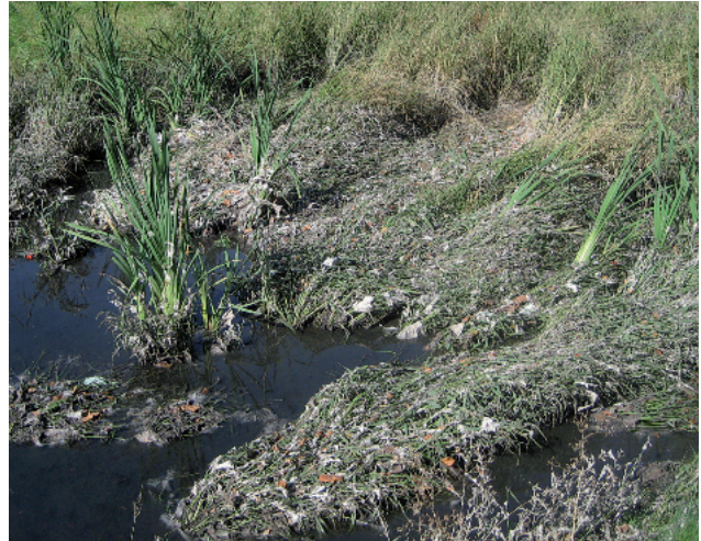
Soil filter without coarse material retention in the inflow area
