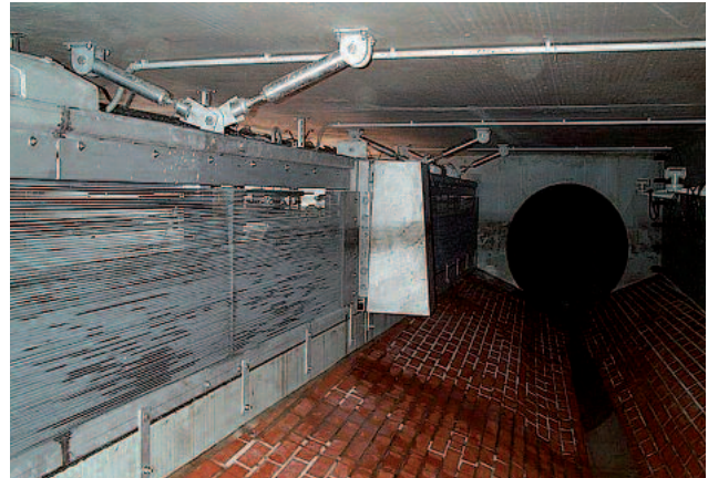
HUBER Storm Water Bar Screen HSW installed at the overflow of a storm water retention sewer
