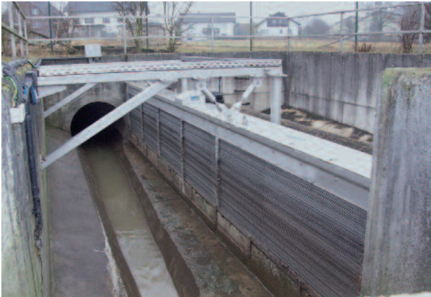
HUBER Storm Water Bar Screen HSW installed at the overflow sill to a storm water overflow tank
