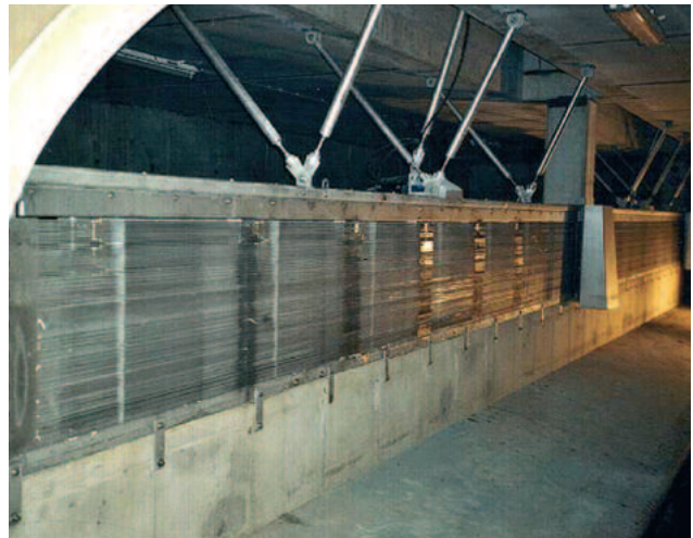
Front view of a HUBER Storm Water Bar Screen HSW installed in a storm water overflow tank
