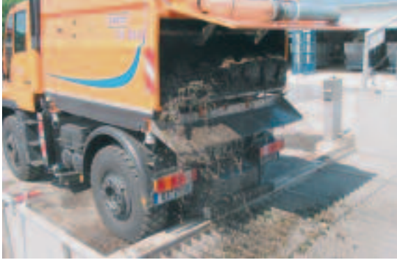
Acceptance tank with bar grate and integrated horizontal dosing screw
