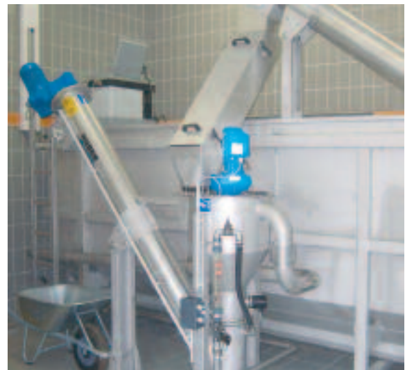
A small Grit Washing Plant RoSF 4/tC washing the classified grit from a ROTAMAT® Complete Plant Ro 5
