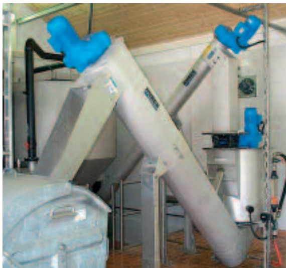
The RoSF 4/t Grit Washing Plant washes the classified grit from a HUBER Circular Grit Trap HRSF
