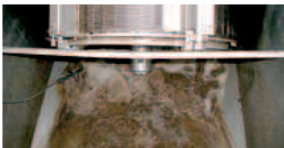
Well-proven wastewater fine screen: ROTAMAT Rotary Drum Fine Screen Ro 2 / RPPS
