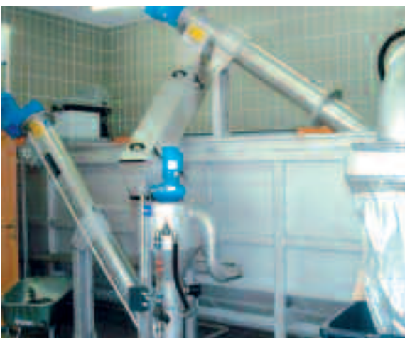
Classifying screw with subsequent Grit Washer RoSF 4/tC
