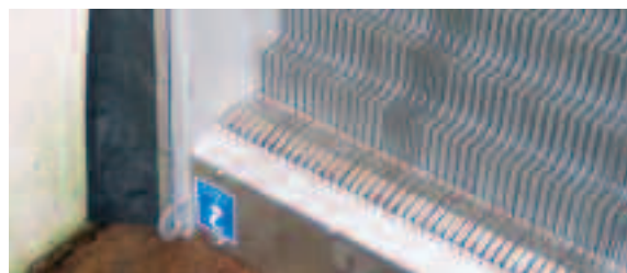
Example of a screen which is suitable for channel installation such that screenings are lifted at bottom level.
